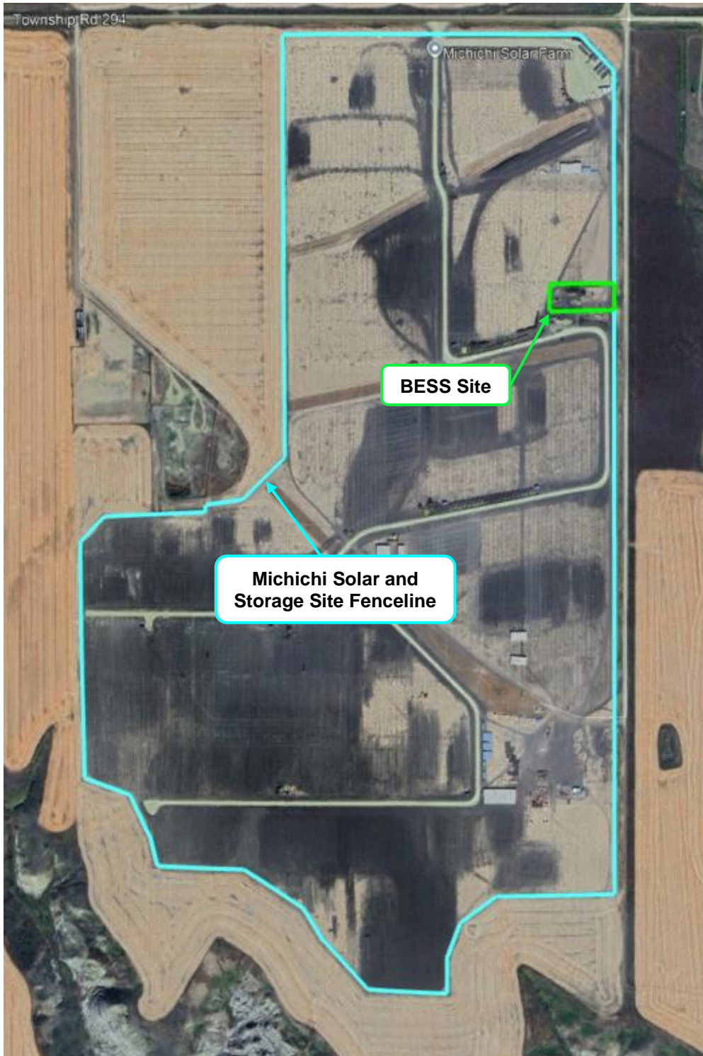
Figure 2 Aerial photograph indicating the Michichi Solar and Storage site fenceline and proposed BESS installation site.
